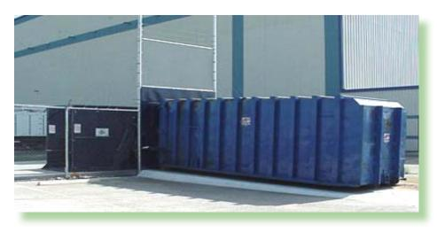
Through-the-Wall/Fence installation, eliminates the need for Security Clearance; the Waste Hauler can switch-out containers from outside the fence area.
